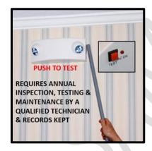
Emergency lighting must be inspected monthly and tested annually. A record must be maintained of all inspection, testing and maintenance. The monthly inspection consists of pressing and holding the test button for 30 seconds and ensuring the lights remain illuminated. The battery should also be checked to make sure the terminals are clean and dry, not corroded, and are firmly connected. If the lights do not work a qualified technician must be called immediately.
